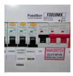
The main thing is to check all of the RCBO are in the up position. If all of them are in the up position press the "Test" button on each one. This will show there is power going down the circuit and confirms the supply to the fuse board is correct and that the issue is inside the parlour/van.
