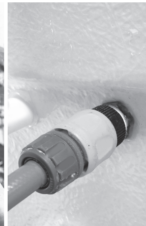
Water supply connection to hydrobath
